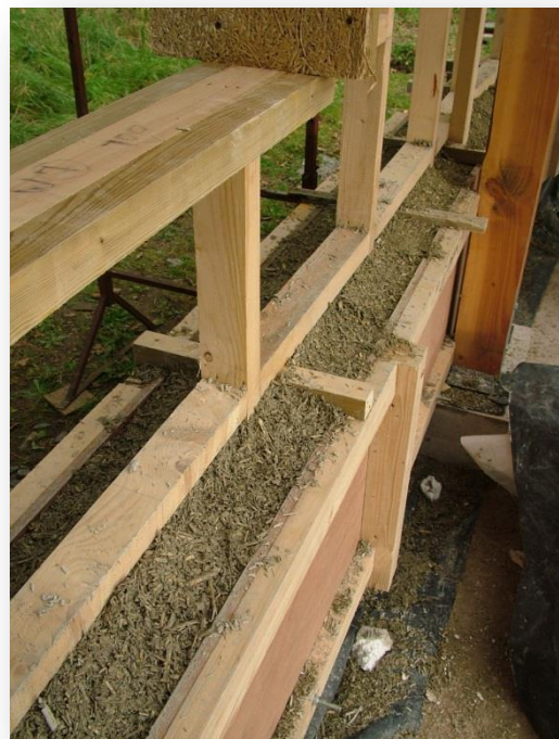
Hempcrete construction in timber shuttering
