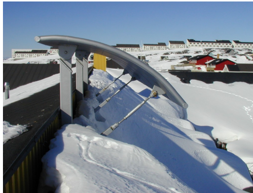
Figure 11: Spoiler at roof at hospital in Nuuk to remove snow by wind
