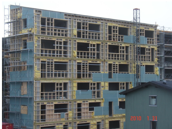
Figure 13: Building in Nuuk, where exterior gypsum boards have blown away
